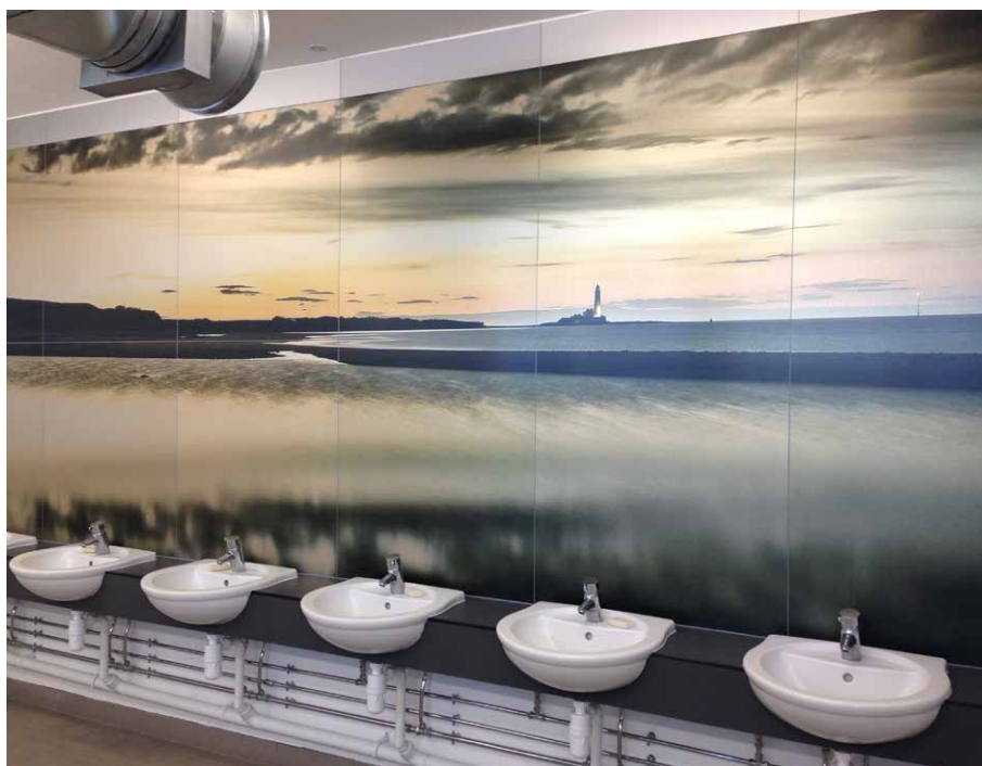
Multitechnic's Anoprinted aluminium is printed on open pore aluminium, then "sealed", creating an extremely durable print to withstand a marine environment.
