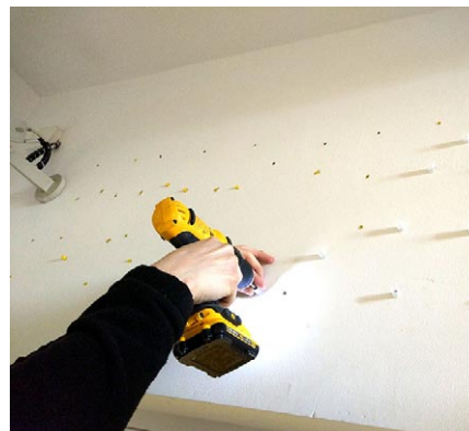
Drill fixing holes suitable for the surface and screw the locators through the template precisely onto the pen marks.
