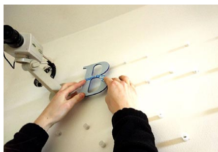
Remove the template and push the letters into the locators fitted to the wall.
