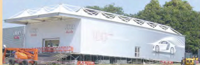
Installation of printed Flex-face to cover marquee 35 x 15 x 6m
