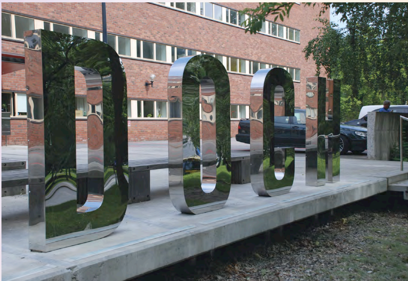
Each 1.7 metre high letter was formed with an internal steel frame which extends below the letter base enabling secure installation through a concrete platform.
