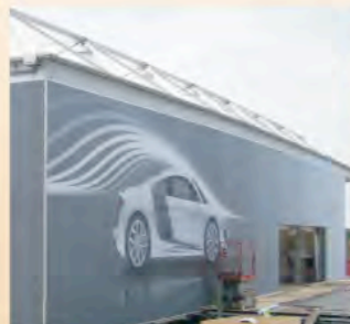
Installation of printed Flex Face to marquee 35 x 15 x 6m
